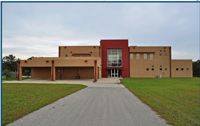
Back View, Office/Research Building
