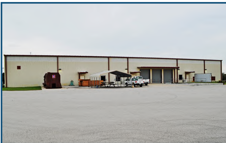
Back View, Manufacturing Building
