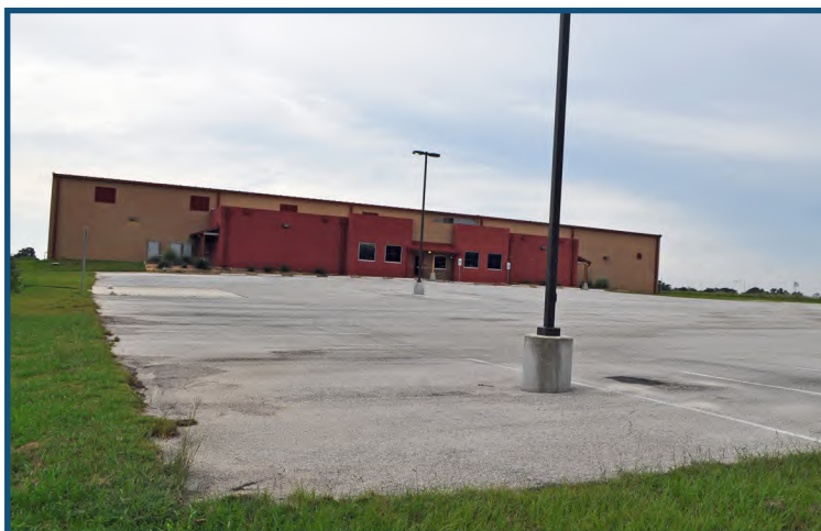
Front View, Manufacturing Building
