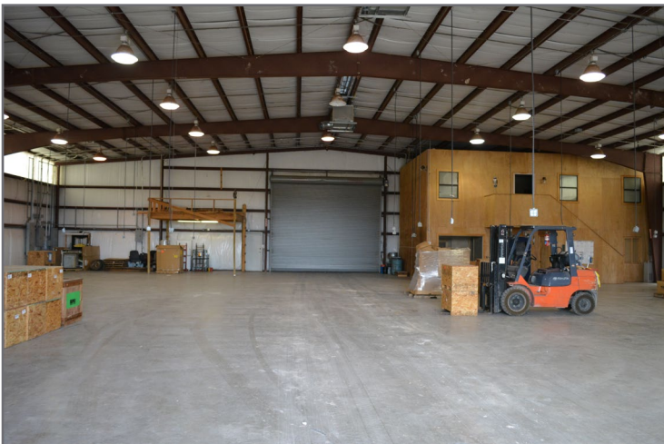
Warehouse, View from OH Door to Front
