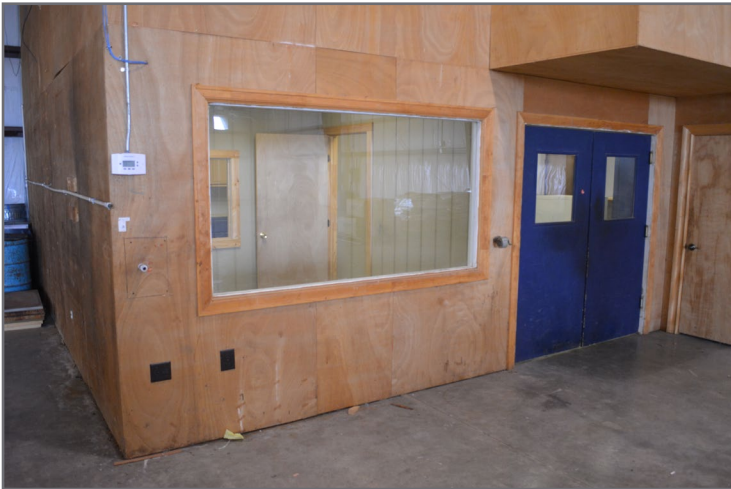
1st Floor Office
