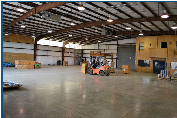
Warehouse, View Rear to Front
