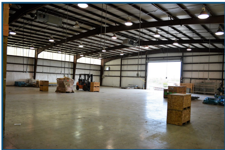
Warehouse, View Front to Rear
