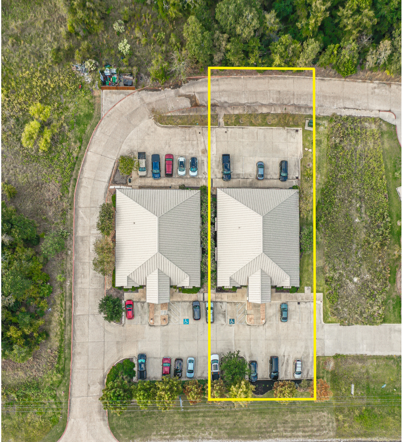
Property lines are approximate
