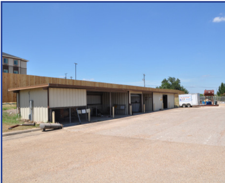
Secure Storage Building
